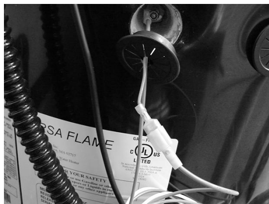
Figure 14 – Wired Low Water Cut-Off Sensor
