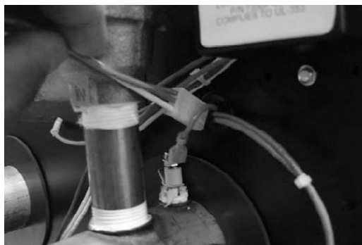
Figure 3 – Routing the 3-Wire Connector
