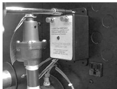
Figure 2 – Attaching the Relay
