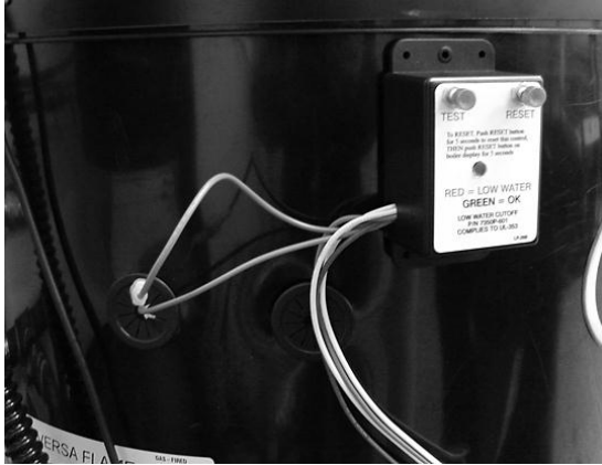
Figure 15 – Relay Installed, Grommet Replaced
