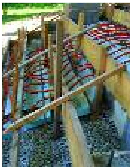
RadiantPEX-AL bends to conform to the shape of outdoor steps for snowmelting.
