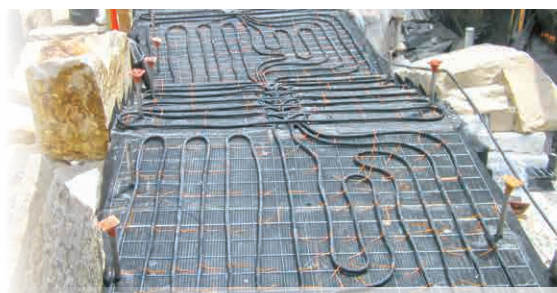
ONIX tubing installation for stairs
